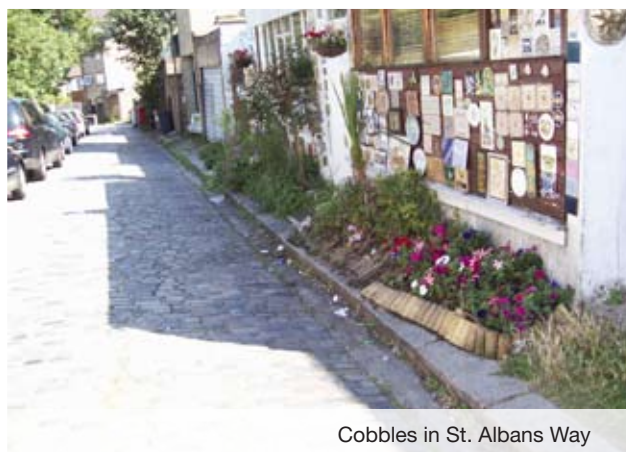
Surviving granite cobbles, Accomodation Road
