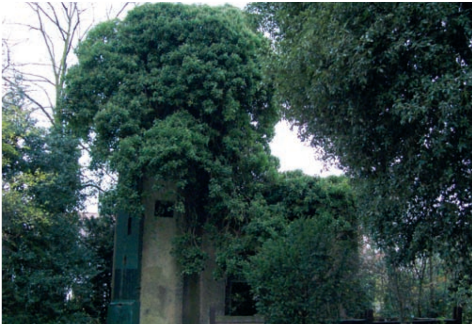
The Water Tower, grade II listed structure at the Avenue House Estate
